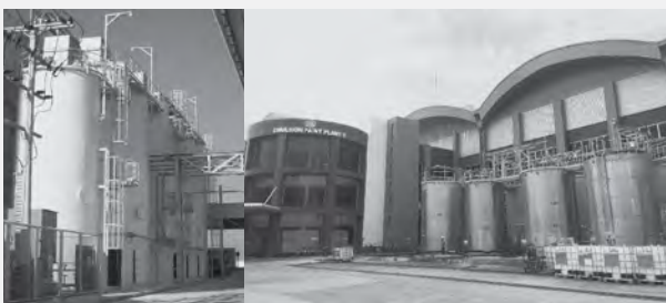
Powdered and liquid raw materials stored in SILO and storage tanks
